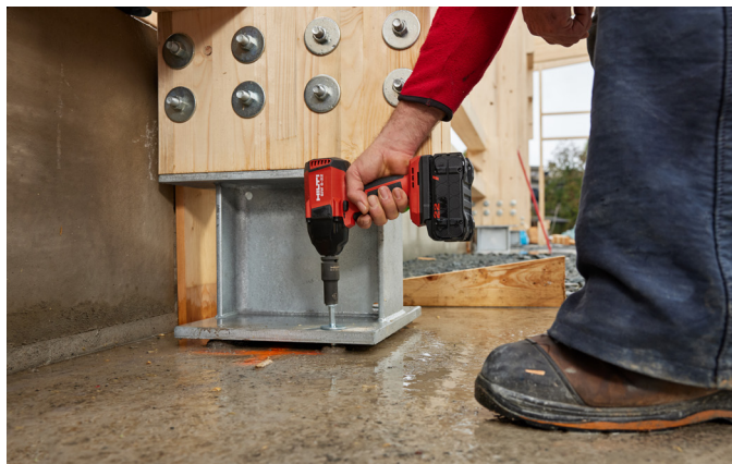
Fig. 2.5: Timber column to concrete application
