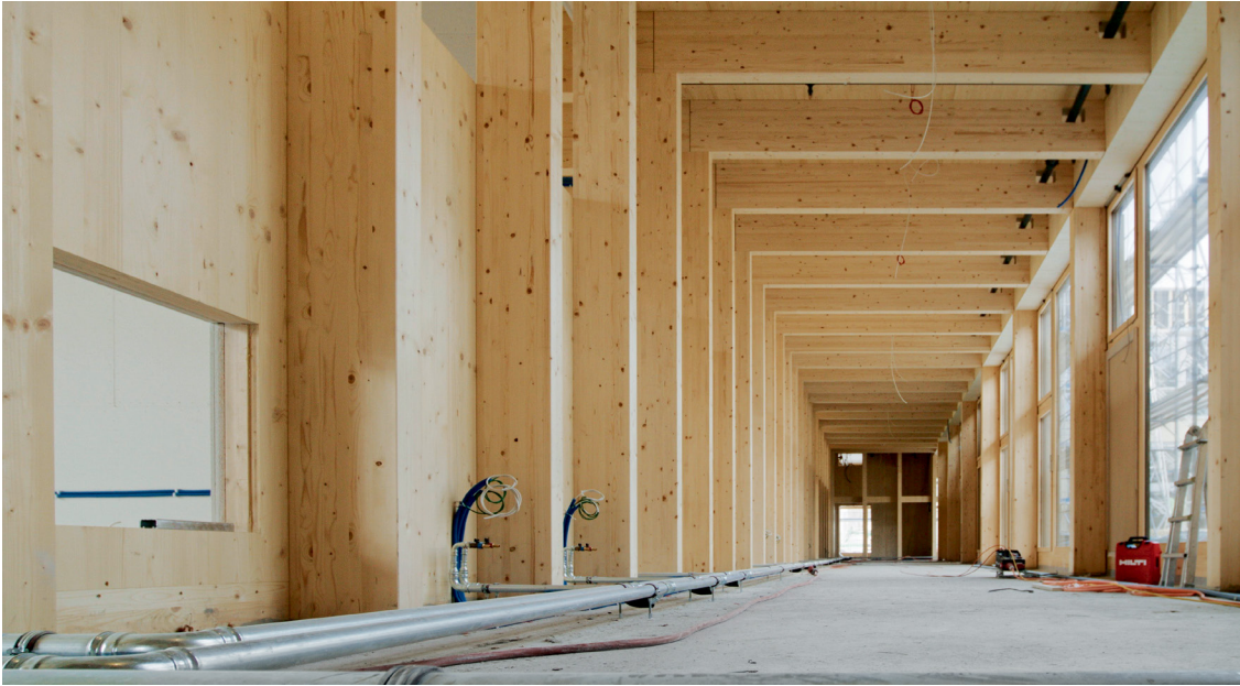
Fig. 1.1: Timber construction site
