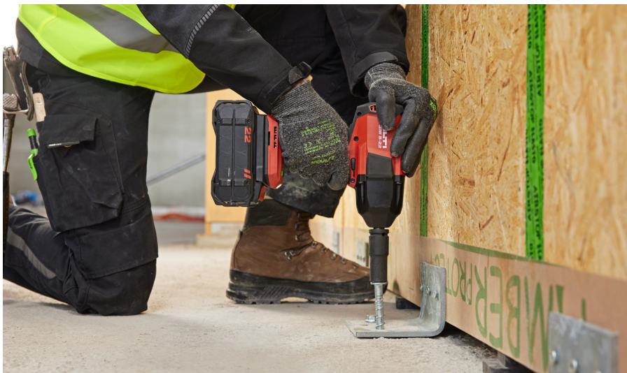
Fig. 2.2: Setting of a concrete screw anchor to fasten a timber frame wall element to concrete via a steel bracket
