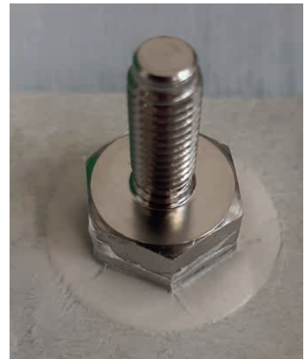
Repaired opening of PFP-coating
