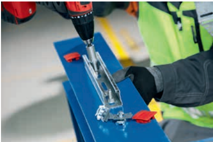
2.1 Pre-drill until shoulder grinds a shiny ring. The drilled hole and the area around drilled hole must be clean and free from liquids and debris.
