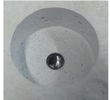
Locally exposed steel with shiny ring after PFP-removal operation
