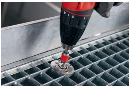
X-FCM, X-FCM-F, X-FCM-R grating discs
